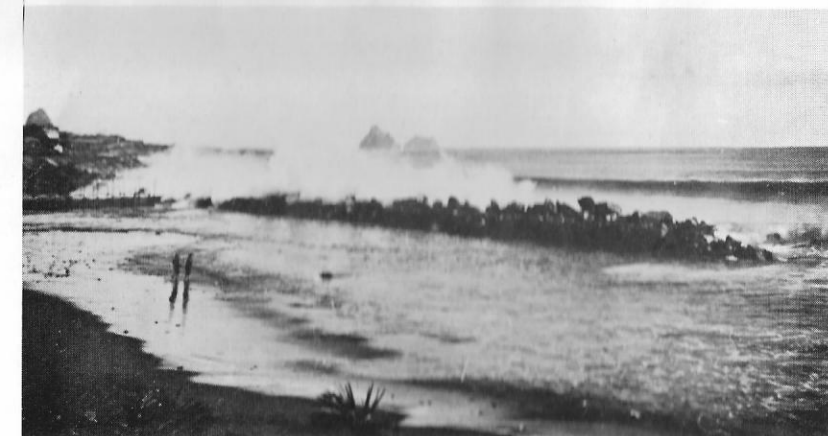
Above: The end of New Plymouth's beach at its front door. This rock wall (under construction) permitted the Railways Department in 1900 to reclaim land and widen its marshalling yards.
