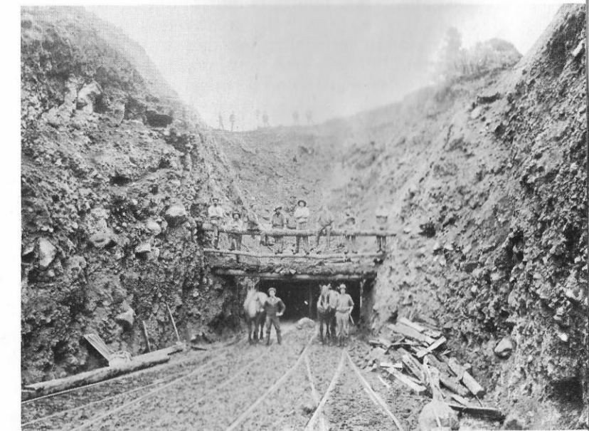
Before the Days of Bulldozers pickaxes and shovels were the only means of digging railway cuttings. (Railways Publicity)
