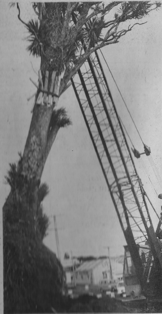
.....the Cabbage Tree was lifted with a crane.
