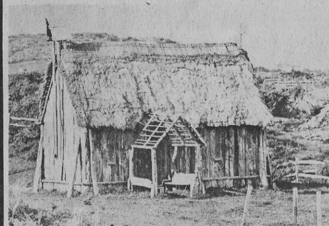
The original Henui Church. This Anglican Church was later replaced by the church pictured opposite.....
